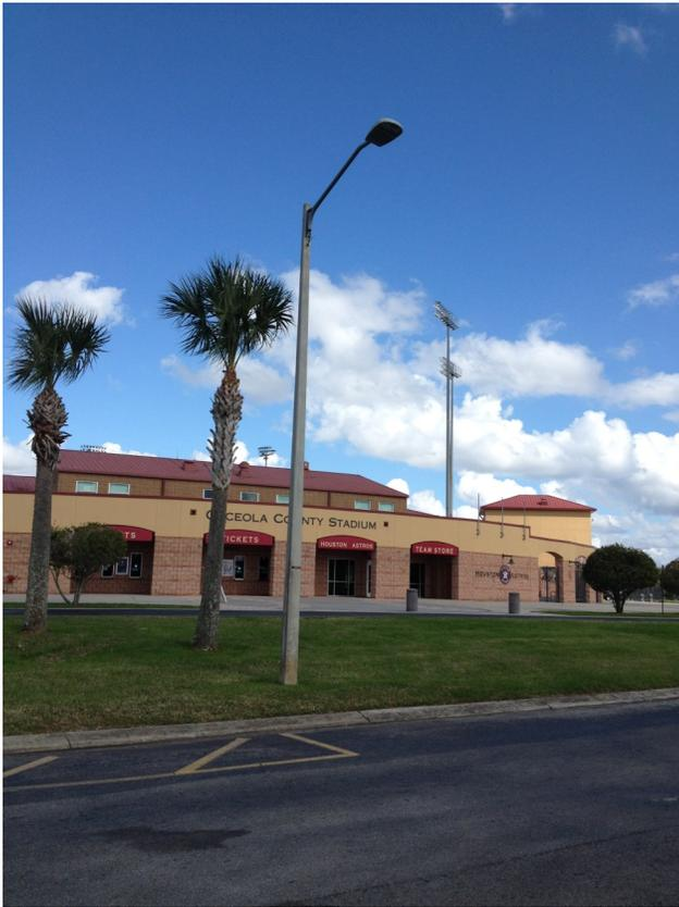
Above: 139w LED Cobra Fixture on 30 ft. Square Concrete Pole. Lease Rate = \$18.02 per month.
