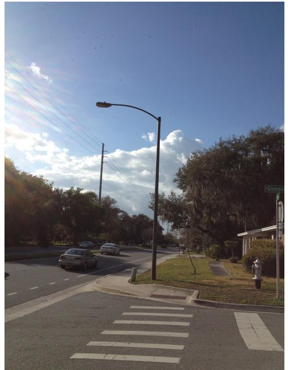
Above: 250w HPS Black Cobra Fixture (full cutoff) on Black Round Tapered Spun Concrete Pole. Lease Rate = \$23.46 per month.
