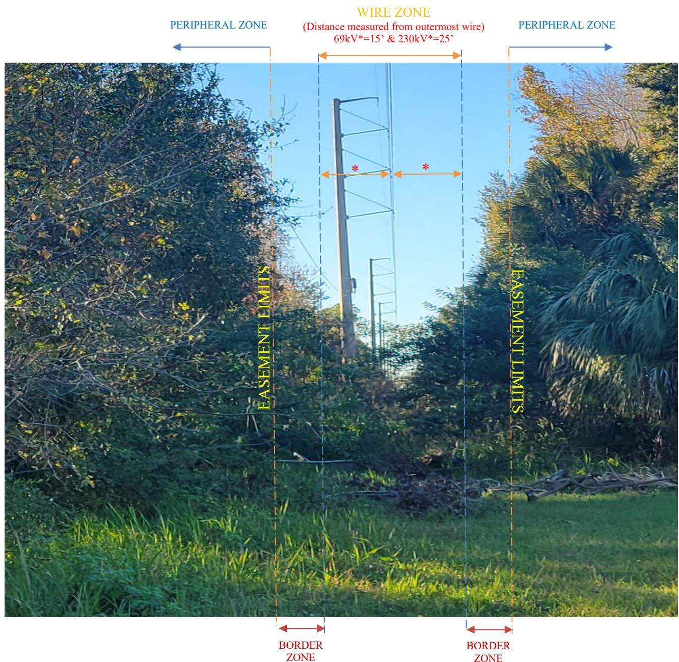
**Wire Zone:** Extends beyond the outermost conductor on both sides. Electrical structure type may vary from single pole to lattice tower or H frame.
