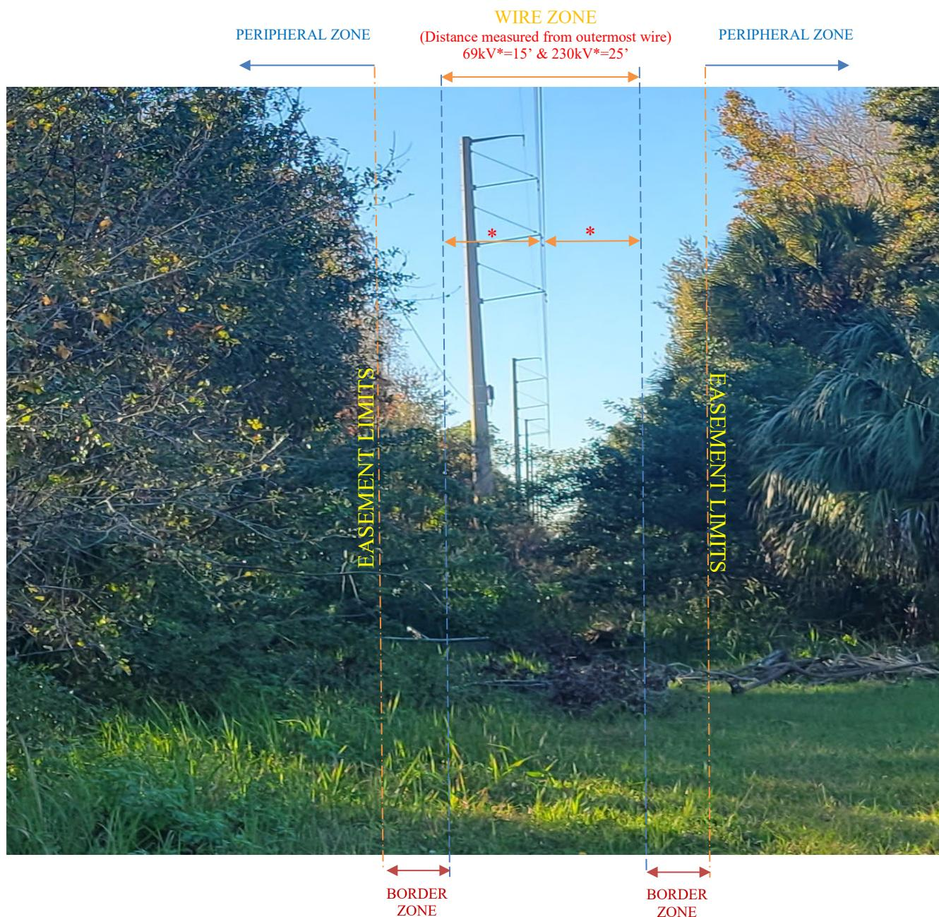
**Wire Zone:** Extends beyond the outermost conductor on both sides. Electrical structure type may vary from single pole to lattice tower or H frame.
