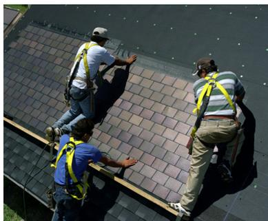
*Thin film solar shingles can replace roofing material.*
